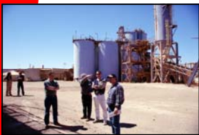
CIP Plant- care and maintenance
